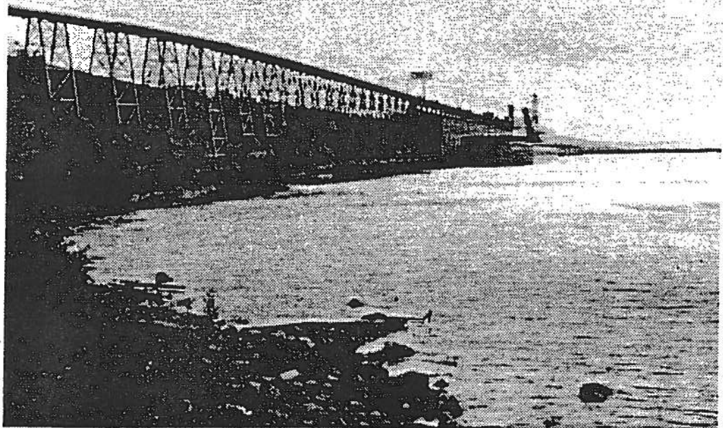
LTV Steel ore docks at Taconite Harbor, Minnesota
